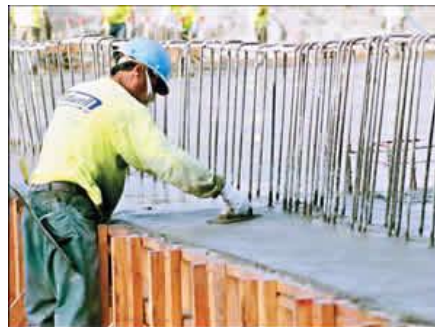
Twenty three million pounds of concrete were distributed over 15 hours—the largest concrete placement in the Coachella Valley to date.
